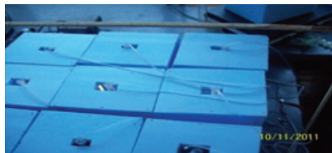
Figure 11. The protective boxes
