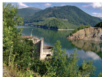
Figure 14. Slipping on the left slope (original photo)
